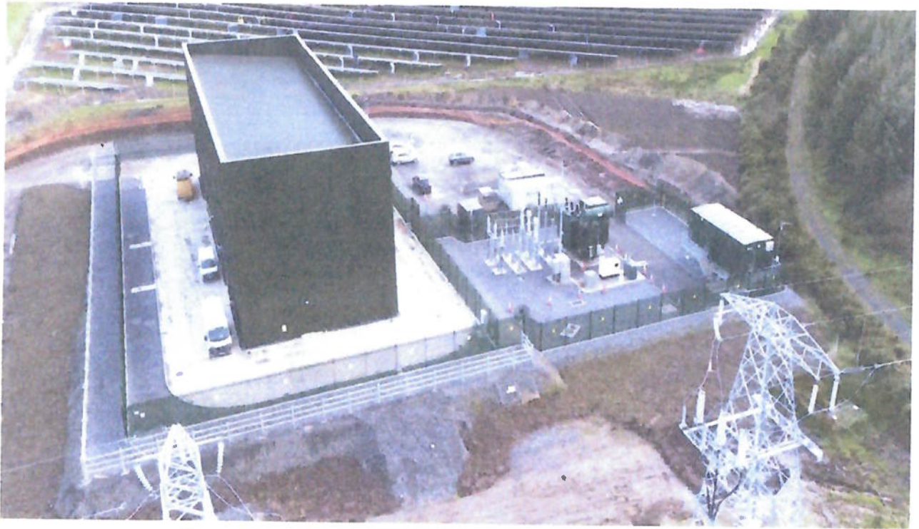
Figure 2-1: Typical 110kV GIS Station Layout (Source: H&MV)
